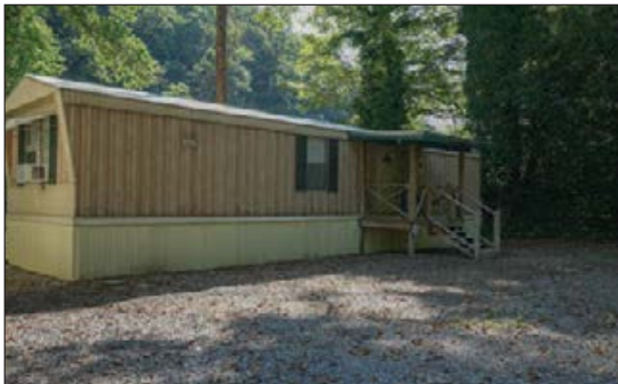
NANTAHALA RIVER! 2 BR 1 bath well maintained home w/ huge screened in porch on the river, carport, storage bldg. Fish, float & swim from your backyard. Close to Nantahala Outdoor Center, Appalachian Trail & Lake Fontana. Call James Mullis @ (828) 338-8585, $12,115 down pmt, APR 4.71%, P&I $1,183.47, $194,000!
