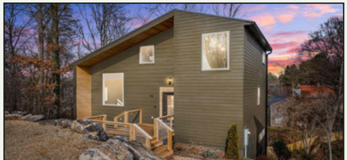
MASTER BUILDER KIRIL NIKOLOV is pleased to present another Quality Build in West Asheville. Three levels of quality construction on a very private West Asheville cul-de-sac. Upstairs we have the Primary Suite, Large Bedroom with En-suite bath complete with soaking tub and shower plus a walk-in closet. 612 sq feet all to yourself! On the main level; open Kitchen/living/Dining with soaring vaulted ceiling, industrial ceiling fan and energy star appliances. Sunny Bedroom and full bath on main as well. Downstairs you'll find an additional 2 bedrooms and full bath. Great for the kids or visitors. All this sited on a large lot complete with your very own natural spring. Fantastic landscaping! $719,000 MLS:4100553 www.rewnc.net/663902 Call Paul Harkrider at 828-458-0844
